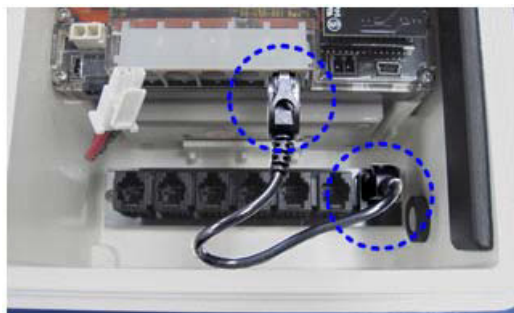
Figure 32: Figure 30: Installing Connector Cable
